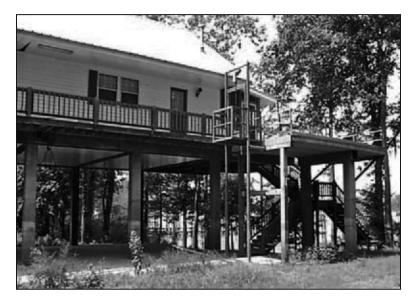
Figure 6-28. House elevated on timber piles
