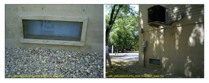
Figure 5E-14. A house where flood openings have been covered by insulation and drywall
